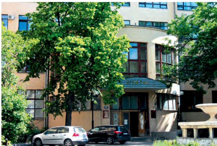
Fig. 1. Building of the Institute of Geology of Ore Deposits, Petrography, Mineralogy, and Geochemistry (IGEM), in whose compass window Ore-Petrographic Museum is situated. Photo: M.K. Sukhanov.
